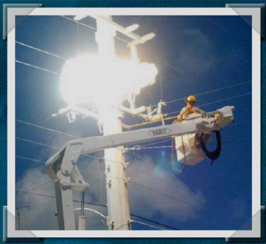
(Worker at the end of a live line tool)
