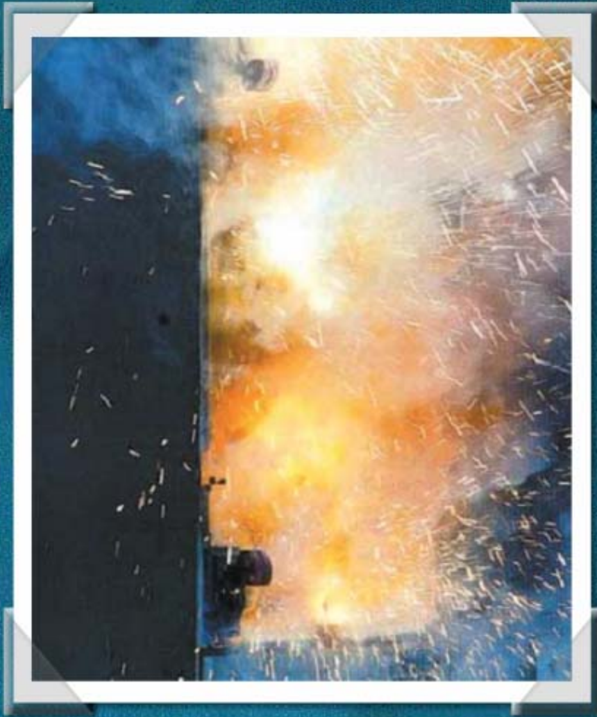
(ARC in a box from a metal clad switchgear)
